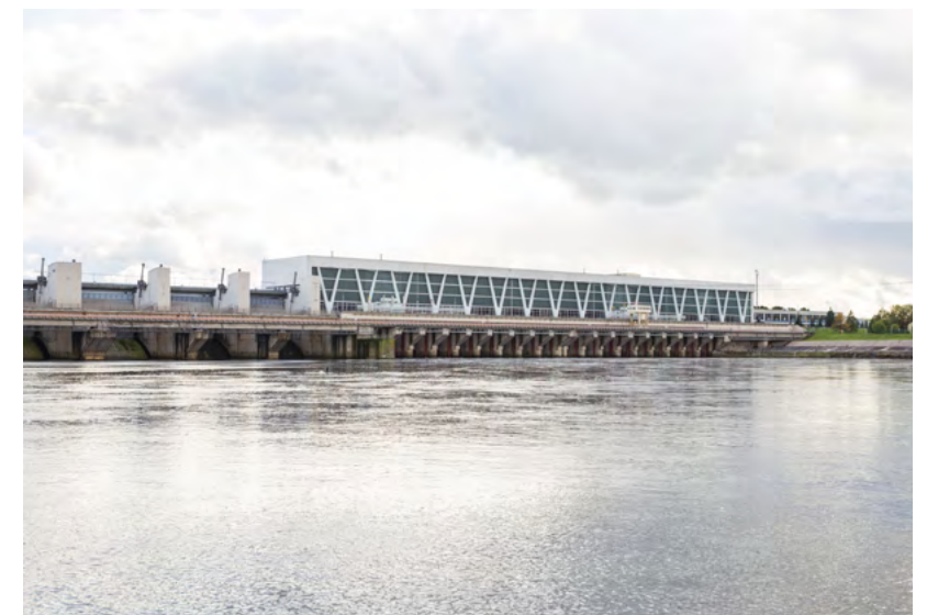
Hydroelectric station on the Daugava river. Photo: Edijs Velciks / Shutterstock.com
